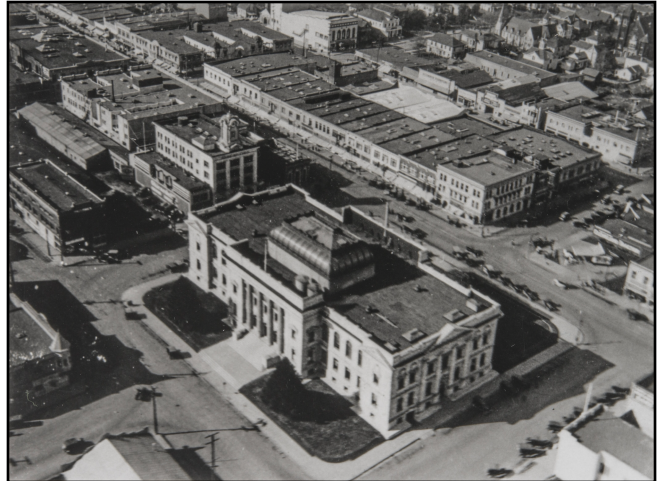
This 1920 aerial photograph of Santa Rosa's Courthouse Square is from the Sonoma County Library Photograph Collection's Gaye LeBaron Historical Photograph Collection, 1871 - 1989 . The Courthouse was dedicated on May 6, 1910 and demolished in 1966.
