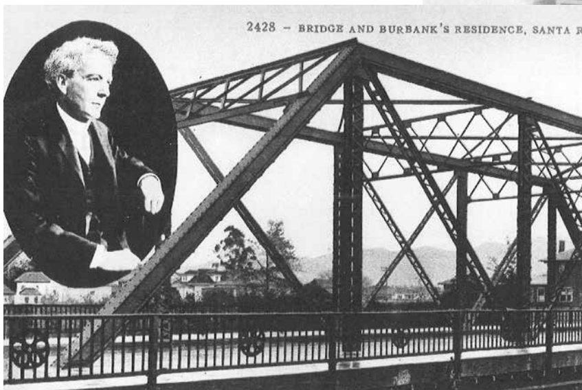
Santa Rosa Creek Bridge and Luther Burbank
