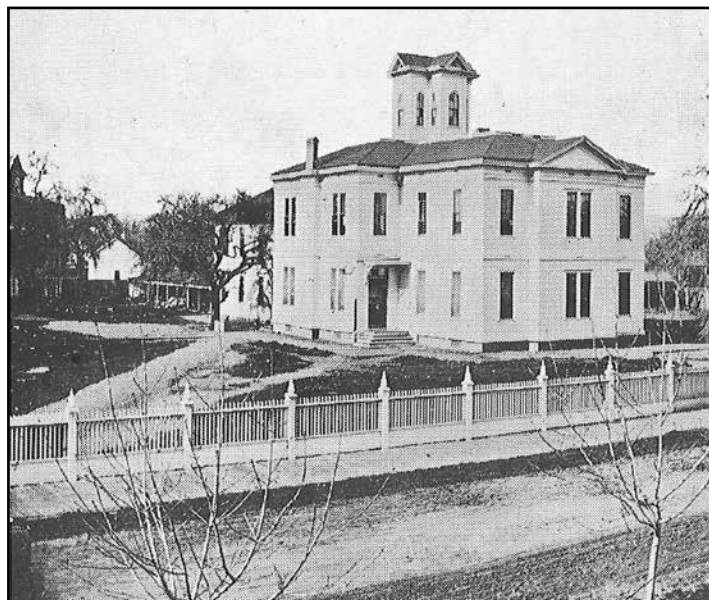
SRHS occupied upper floor Fourth Street School Santa Rosa High School Museum
