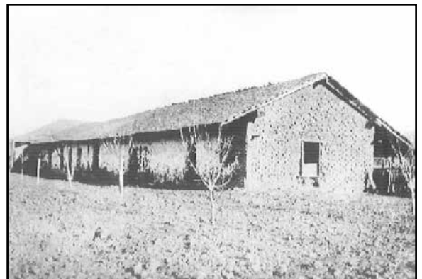
The Carrillo Adobe, ca 1930s
