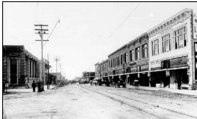
View of 500 Block of Fourth Street, 1907 Sonoma County Library Collection
