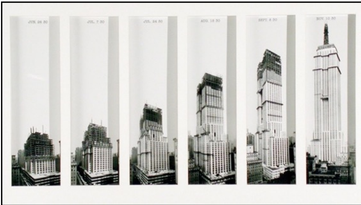
Construction phases of the Empire State Building. Shown: June 26, 1930 through November 10, 1930 History.com
