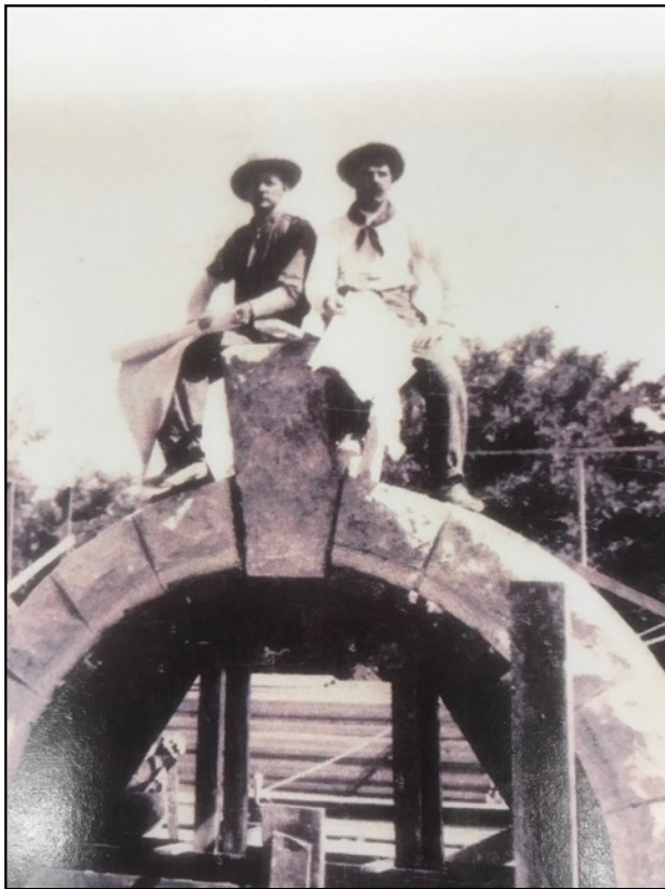
Italian stone masons sit atop an entrance arch during construction, Circa 1904 Sonoma County Library Collection
