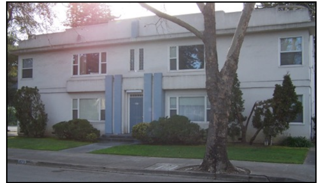
Apartment building at 825 Washington Street today, built 1948
