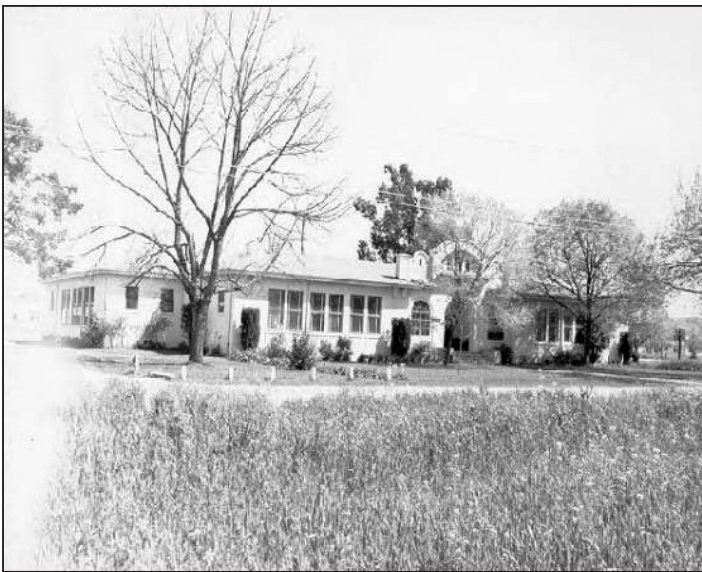
A number of stores now fill the field across from Lewis School Sonoma County Library
