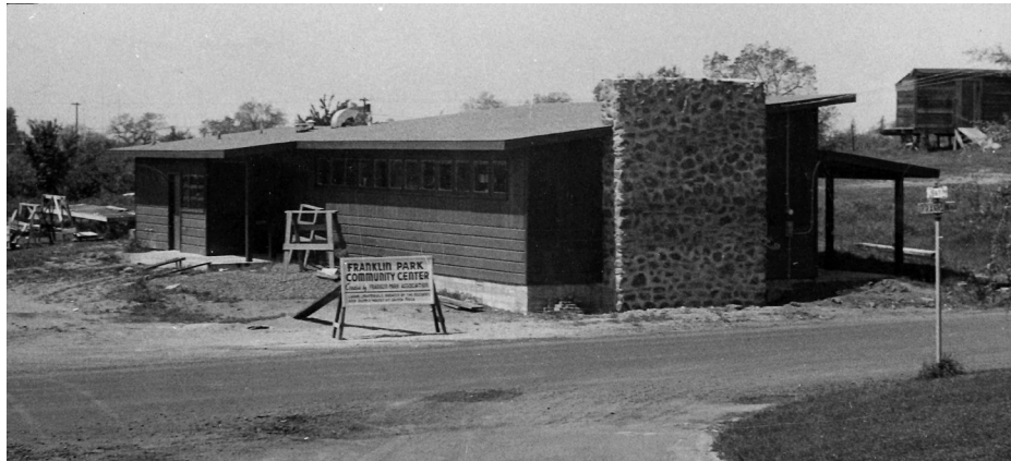
An almost finished clubhouse proudly sits on Franklin Avenue Franklin Park Association Archives
